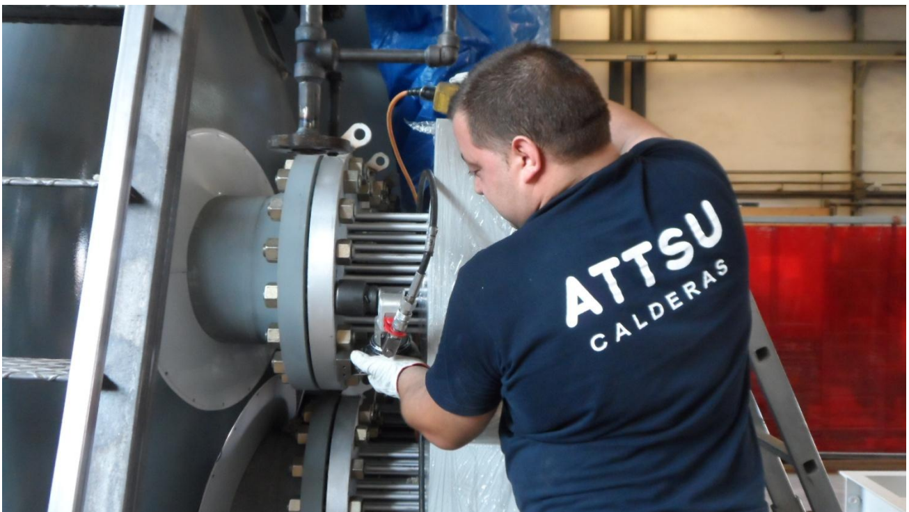
RESISTANCES ASSEMBLY USING A HYDRAULIC TORQUE WRENCH
