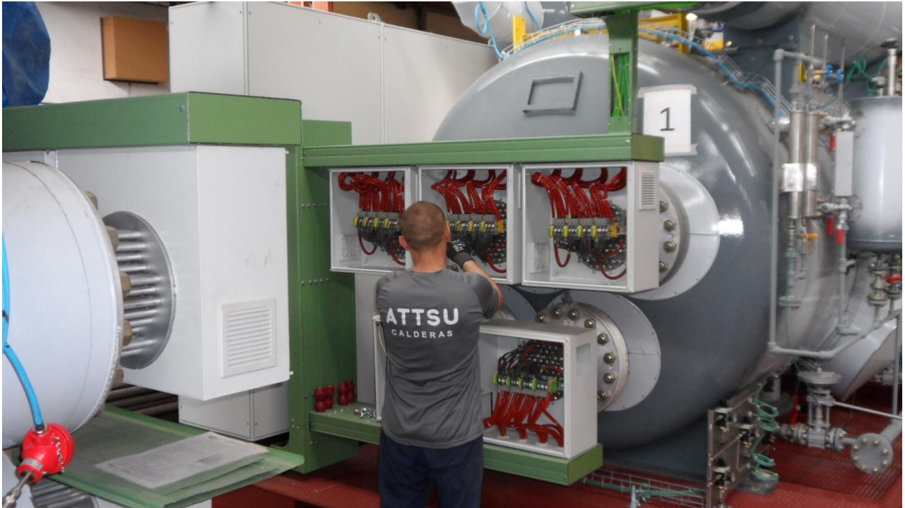
GE-4600 – HEATING RESISTANCES CONNECTION (3 MW ELECTRIC POWER RATE)
